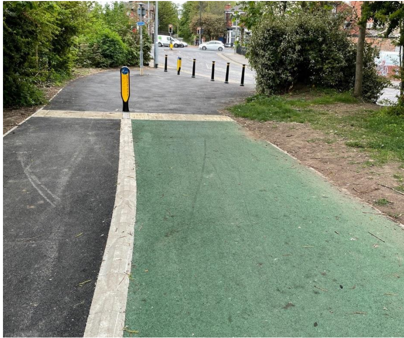
Example of green coloured surfacing on Hull to Cottingham route
