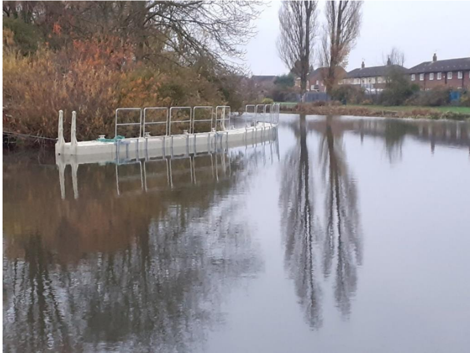
Figure 1 Jetty moored off island
